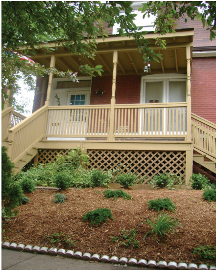
Rebuilding Together home on Gibson
